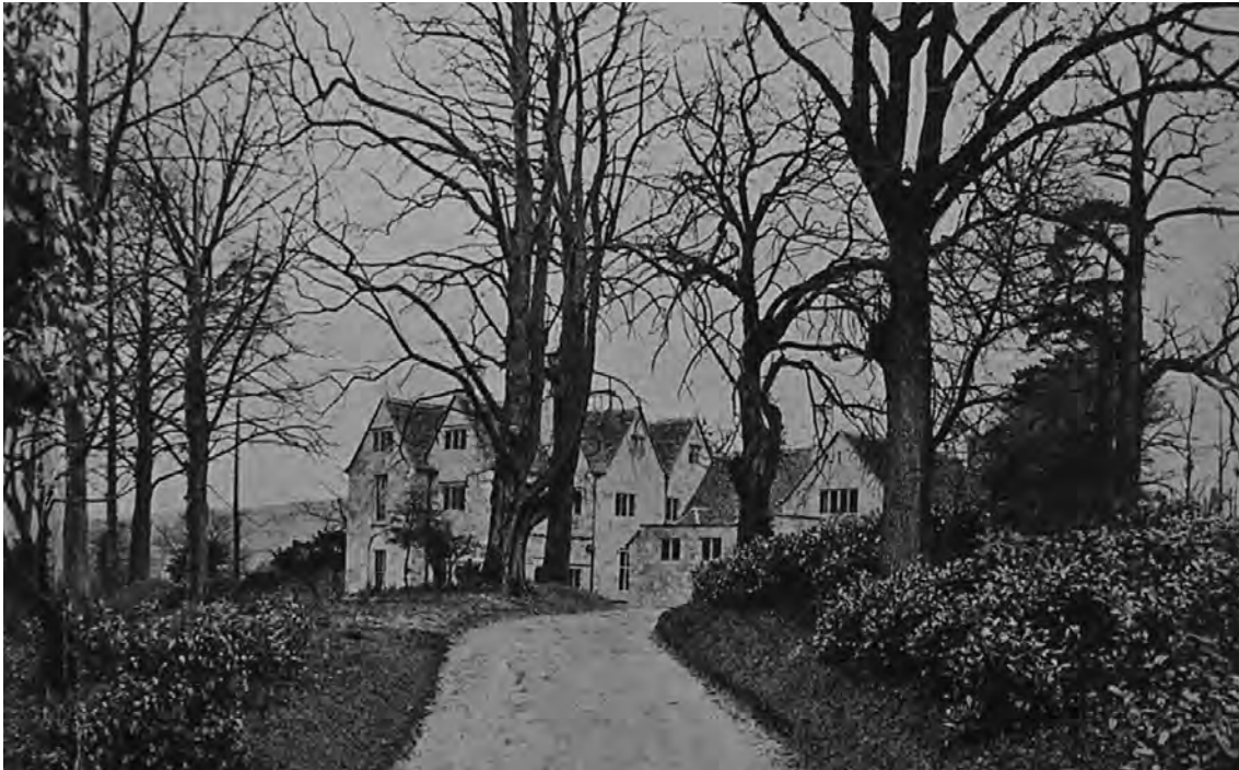
The new drive to Lullingworth
