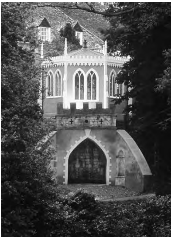
The Eagle House after the rebuilding of the missing superstructure
