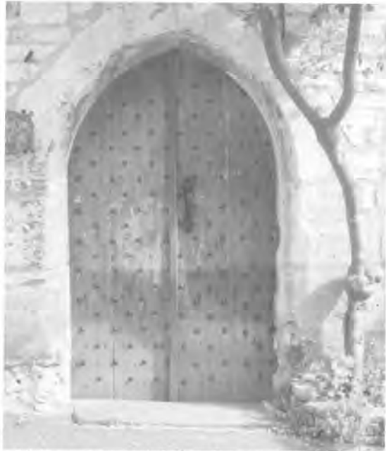
14th century pack horse doors in Bisley Street leading to clothiers yard
