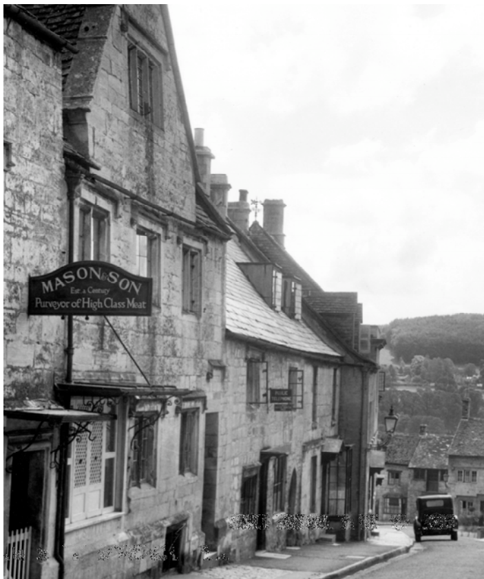
Second Telephone Exchange Bisley Street
