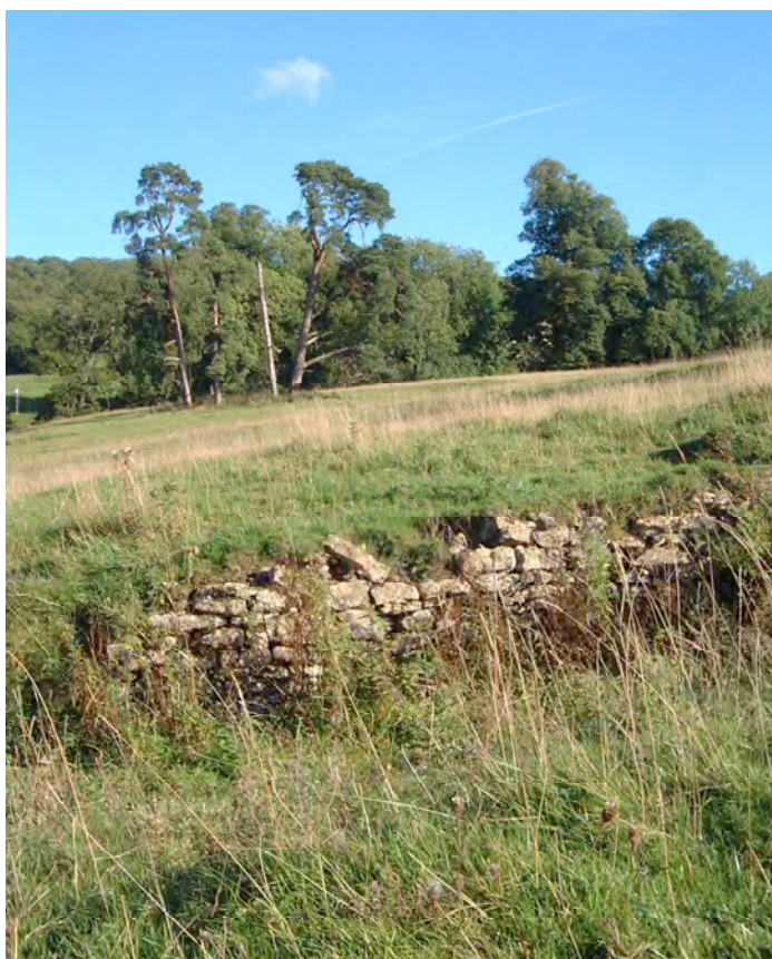
Remains of ha-ha and landscape garden below Brownhill Court.
