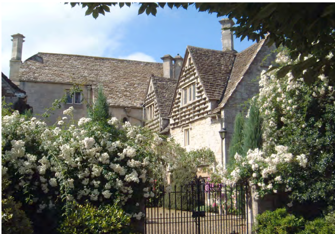
Sheephouse dovecote in gable.
