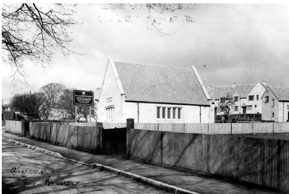
First purpose-built Telephone Exchange, Pullens Road
